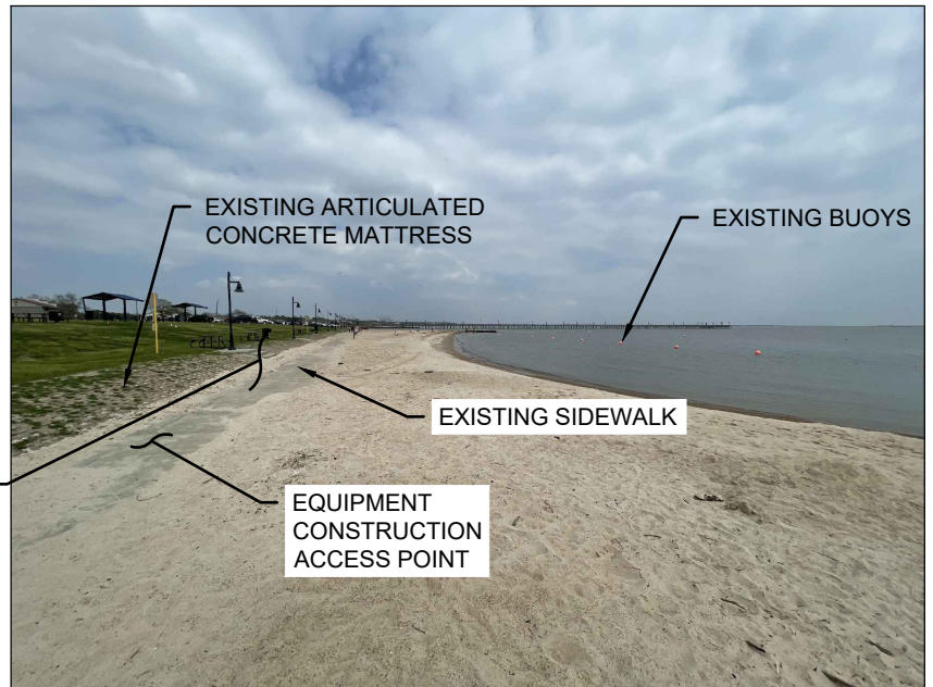
SYLVAN BEACH SOUTH CELL FACING NORTH
